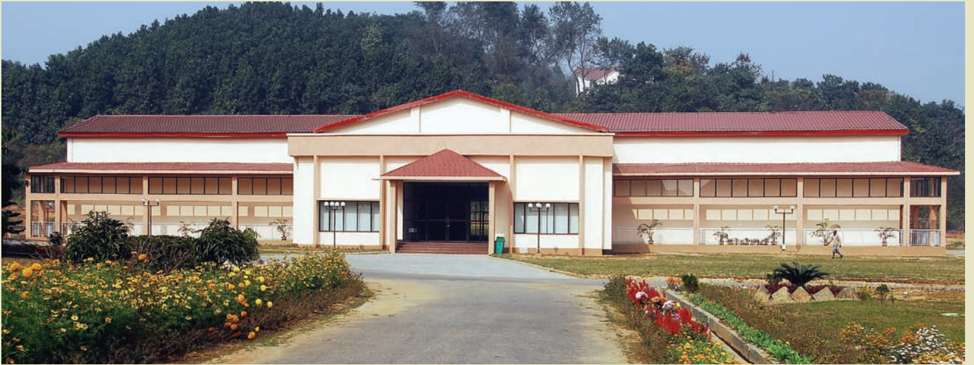
The new Conference Centre with four halls and a utility space has recently become functional.
